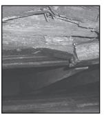
Standing water creates excessive humidity. Unless this is removed and the area kept dry your foundation will start to deteriorate and thus move up into other areas and continue the deterioration process. Mold and mildew are common occurrences in these
