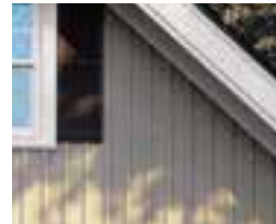
Board & Batten are vertical panels with a rugged look
