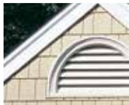
Shakes are square-edge shakes with the look of hand-cut cedar
