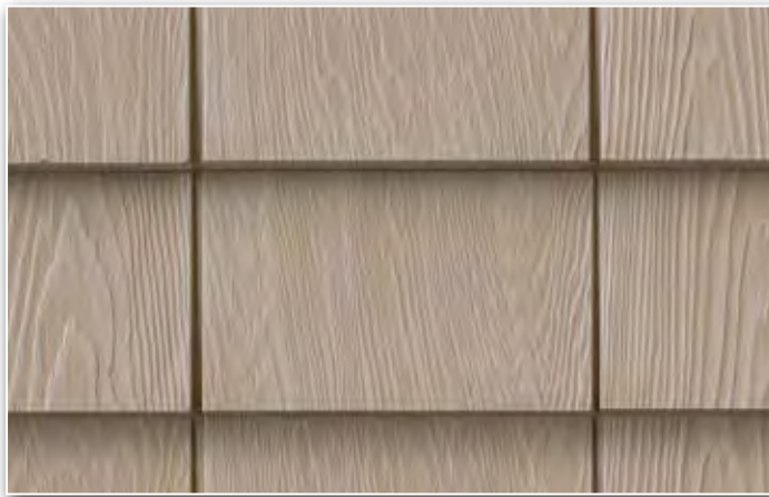
Incorrect Installation
