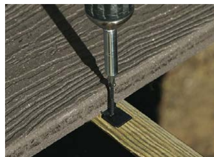
Hidden Fastener Installation to Joist
