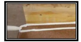
Move the flashing into position behind the house wrap material and over the decking assuring that the sealant is bonded to the decking and flashing.
