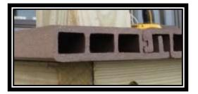
Position the first board to the deck with the fastening wing to the right side with the board overhanging the installed fascia board 9/16".
