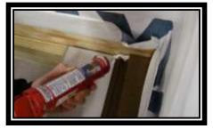
If the length of the board will be placed along a wall of the house also place a bead of sealant on the joist where the board will rest.
