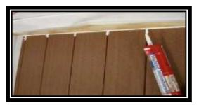
Cut and position coated aluminum (or other material) flashing with the flashing being install behind the house wrap material and over the decking.
