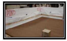
Seal the flashing to the wall under the house wrap using a sealing tape to assure that any moisture that penetrates the house wrap will not find its way behind the flashing.
