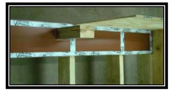
Seal the pan to each protruding post with a waterproofing butyl seal tape. Seal carefully to the aluminum pan and up each post on all sides at least 3". Assure that the seal is tightly adhered to all surfaces.
