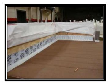
Turn the house wrap material down over the flashing and seal the house wrap material to the flashing with a sealing tape.
