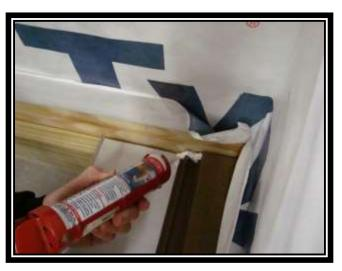
If the length of the board will be placed along a wall of the house also place a bead of sealant on the joist where the board will rest.
