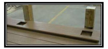
Position the prepared perimeter board over the "through the deck support posts" and position it to the deck with the perimeter board wing over the installed first board allowing a 3/16" gap between the perimeter board and the deck board.
