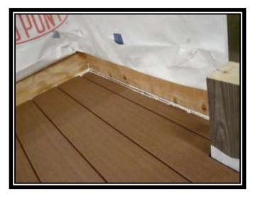
Assure that the deck board is properly positioned and that the second deck board will fit within the pan at the up turned lip when it is installed.
