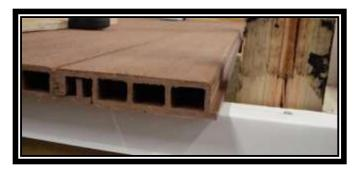
Cut a 1/4" wide kerf the entire length of the top surface of the final board and 1/4" from the wall that has just been altered.
