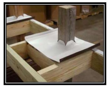
Place a bead of sealant along the back edge of the water diverting pan to form a dam that will help assure that water will not flow backward and will not find its way to the area below. Provide blocking under the pan to provide support.
