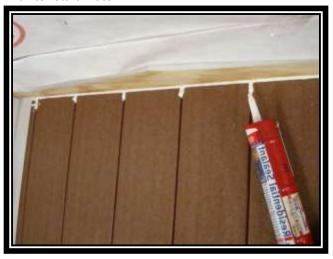
Cut and position coated aluminum (or other material) flashing with the flashing being install behind the house wrap material and over the decking.
