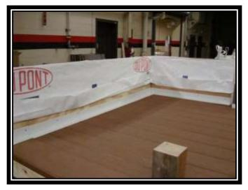
Seal the flashing to the wall under the house wrap using a sealing tape to assure that any moisture that penetrates the house wrap will not find its way behind the flashing.
