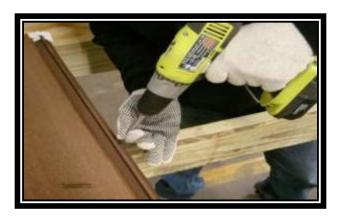
Step B-2: Prepare and Install Left Side Perimeter Board (From GeoDeck Commercial Board)
