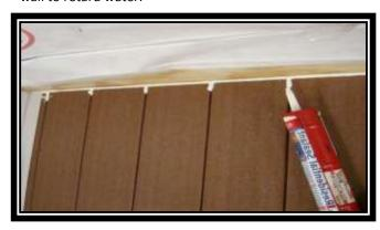
Cut and position coated aluminum (or other material) flashing with the flashing being install behind the house wrap material and over the decking.
