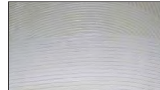
Example of properly troweled adhesive application
